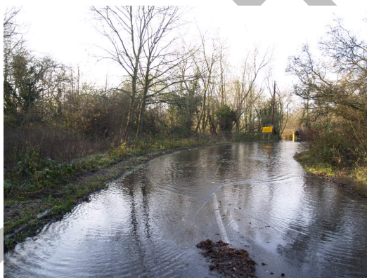
Figure 6. Flooding of Sandford Lane in 2009.
