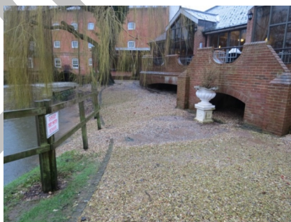
Figure 1. An image of water along Mill Lane almost reaching the Moat House Hotel.
