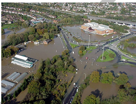
Figure 2: Loddon Bridge roundabout
