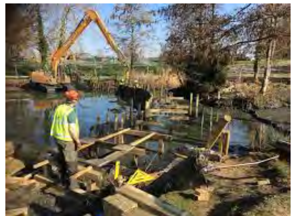
De-silting and boardwalk construction
