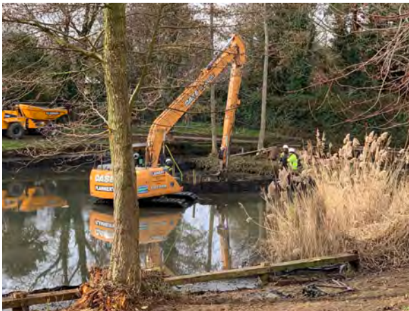
De-silting and boardwalk construction
